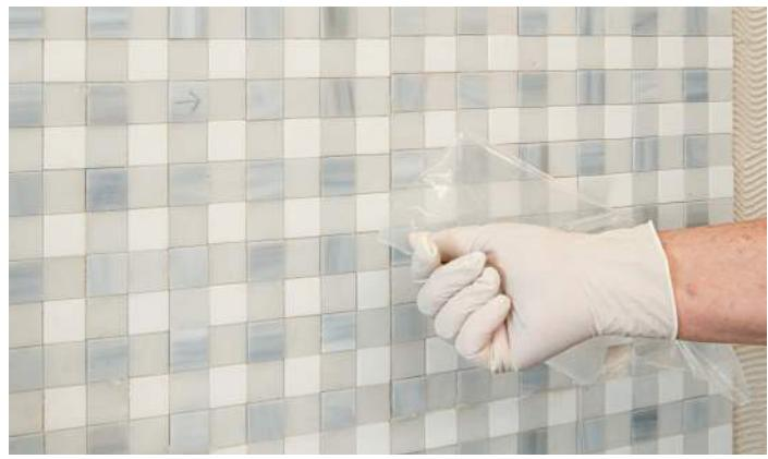
**Step 5** To achieve the flattest possible surface, lightly tap the sheets using light pressure with a grout float or a wooden beating block and a mallet. To unify sheet transitions, tap from one sheet to the next.
