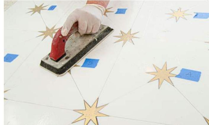
**Step 4** To achieve the flattest possible surface, lightly tap the sheets using light pressure with a grout float or a wooden beating block and a mallet. To unify sheet transitions, tap from one sheet to the next.
